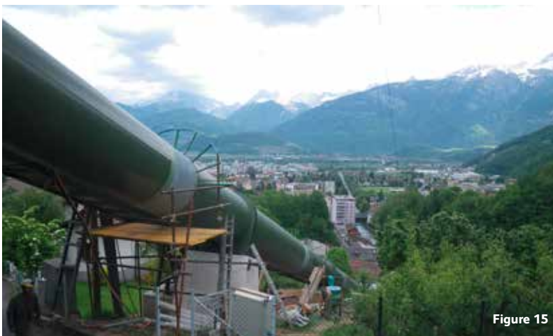
Evaluation of corrosion protection on a water pressure pipe
