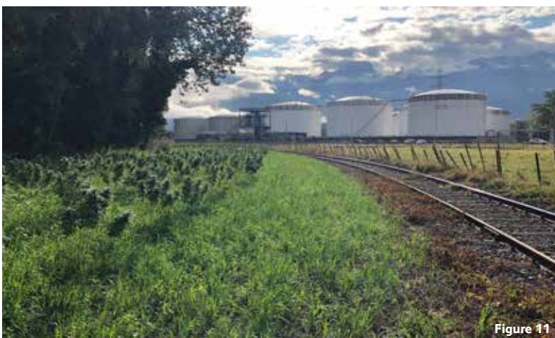
Corrosion investigations in a tank installation
