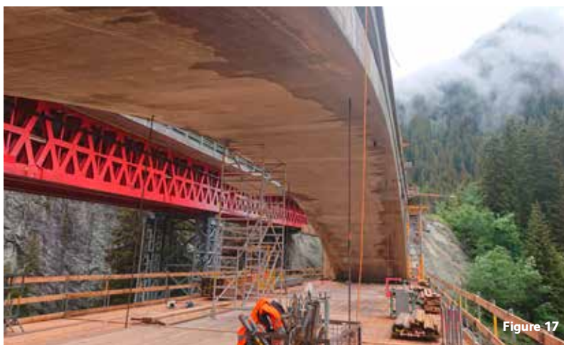
Condition assessment of a reinforced concrete bridge
