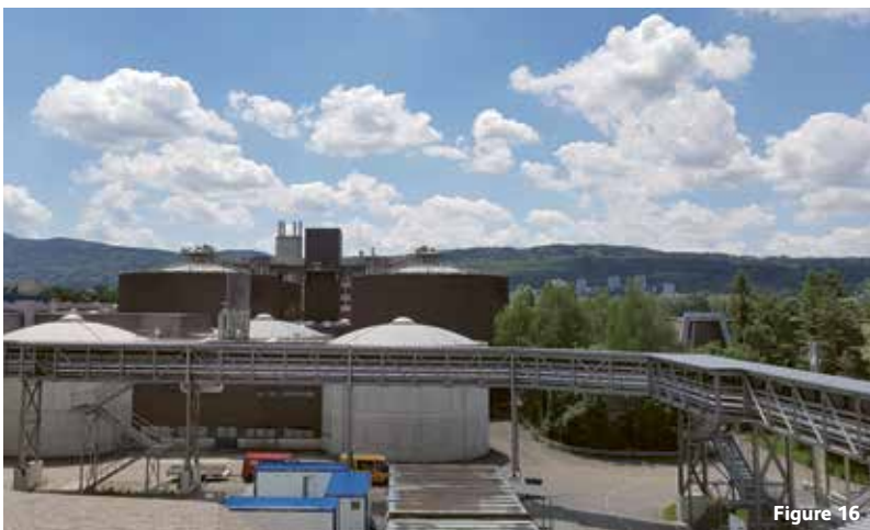
Checking the corrosion protection in a sewage treatment plant
