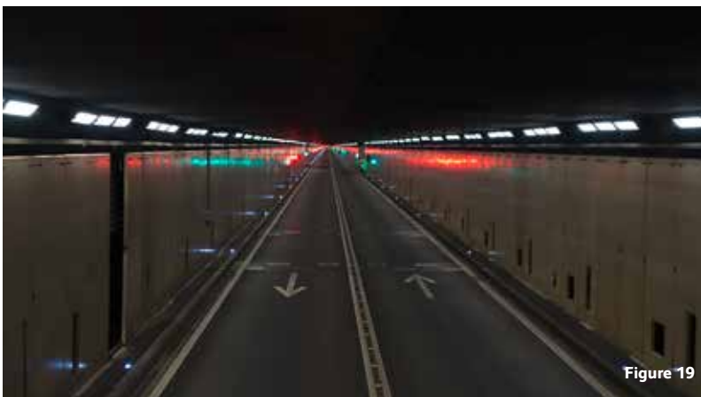
Corrosion investigation on the intermediate ceiling of a road tunnel
